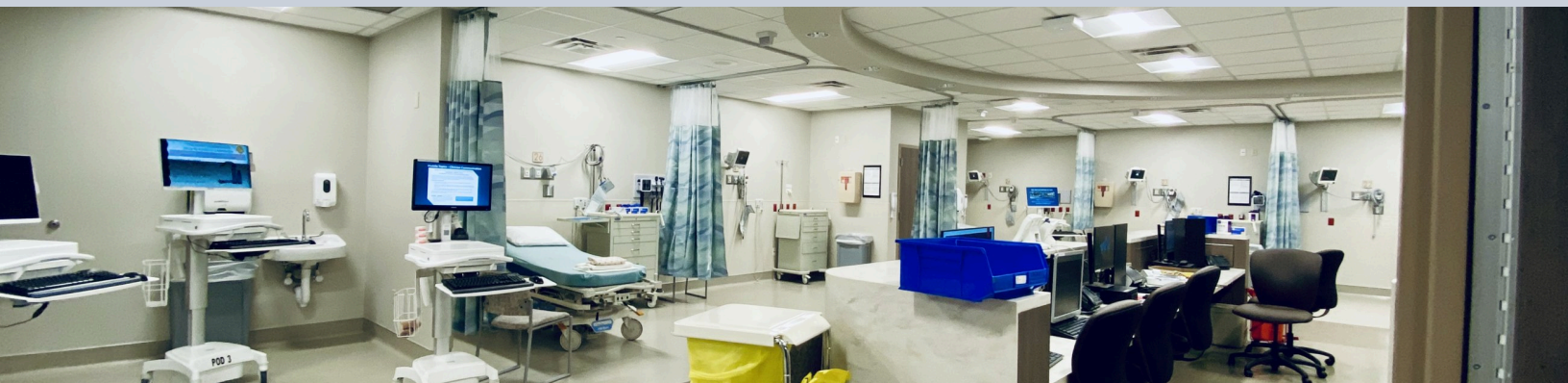
Baptist Medical Center emergency department renovation, San Antonio, TX · GC: Robins & Morton
